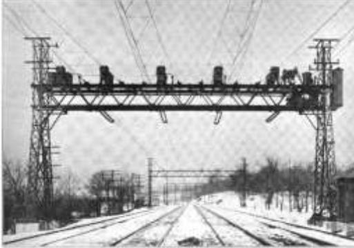
Four-Track Arthur Bridge with Circuit Breakers and Section Breaks.
